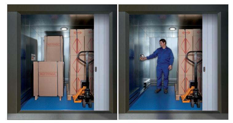
Conventional goods lift mode. The load can take up more space, and the lift is operated from the button displays on the different landings, requiring the presence of an operator on each floor or one moving between landings externally.
